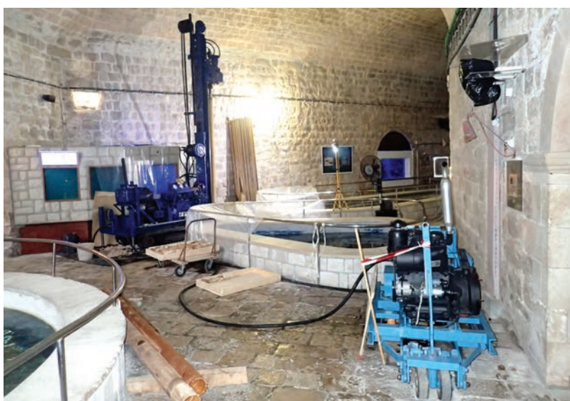
Figure 10. Construction of a borehole in 2016 for pumping sea water into the aquarium from the ground below the fortress (Photo by V. Kožul).
